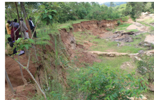
Figure 23: An area affected by flooding in Tambua Ward
